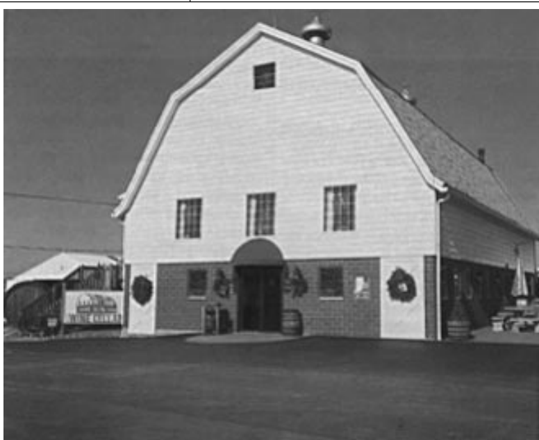
Shown above is a good example of how to reduce the risk of accidents in the parking area of a roadside market. This clean and smooth asphalt parking lot covers a large area near this winery shop and slopes gently up to the entrance, eliminating the need for steps. The entrance way is also well-maintained
